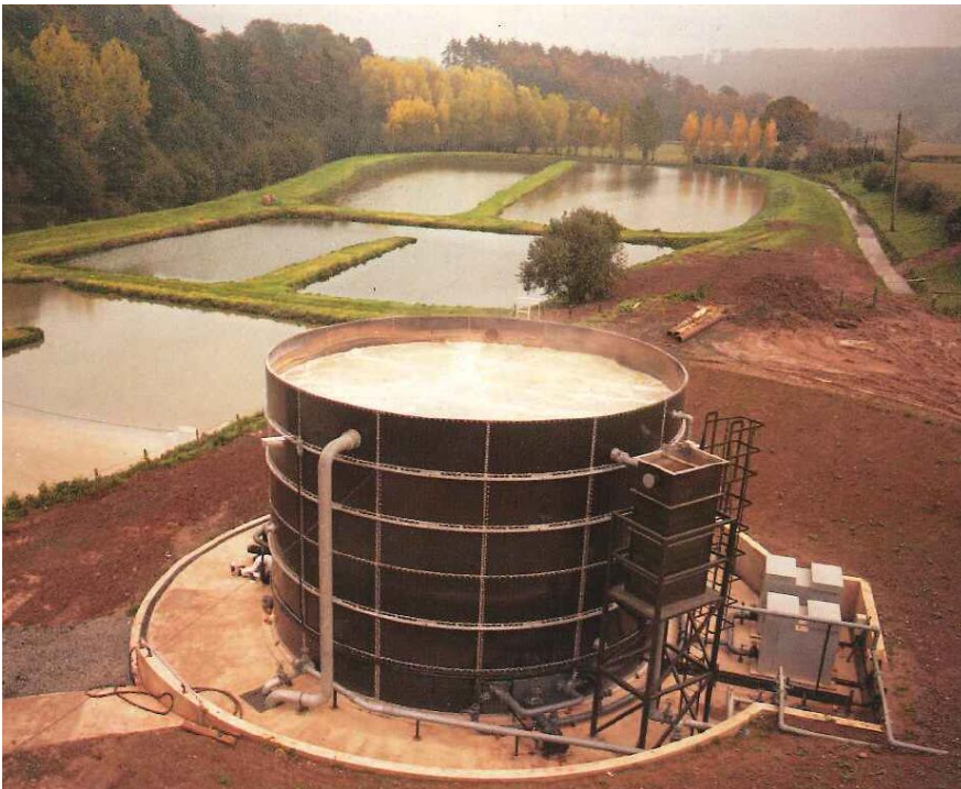
High intensity aerobic reactor using VO 2 aerators at Cadbury
