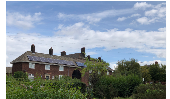
Photovoltaics on a residential property
