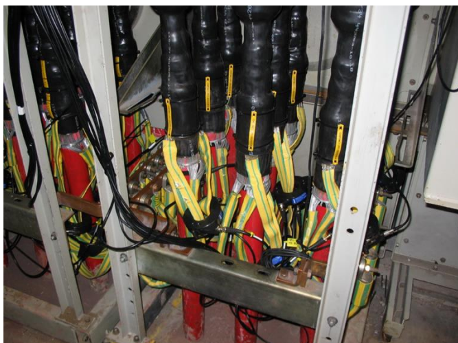
Figure 3 RFCTs Clipped Around the CHP Cable Screen Earth Terminations
