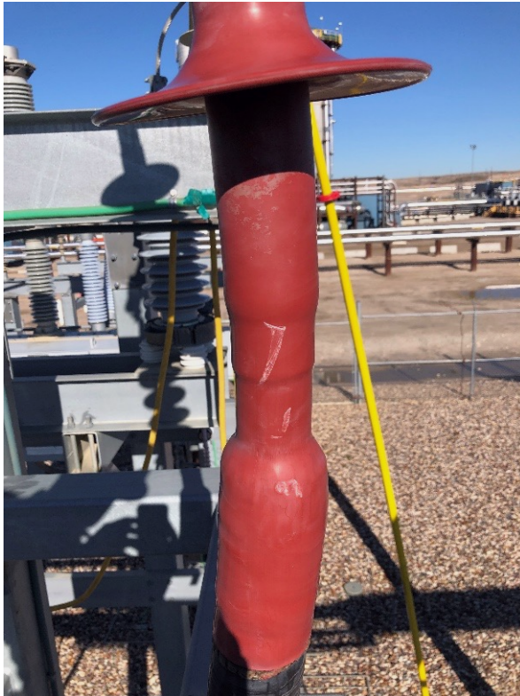
Cable termination H3 after cleaning
